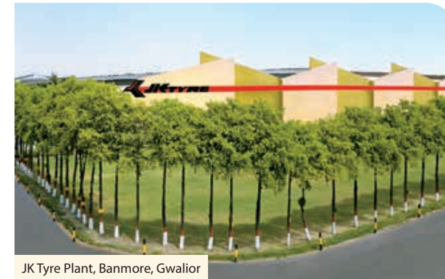
JK Tyre Plant, Banmore, Gwalior
